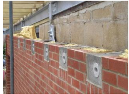
Schwegler 25s installed in brick wall
