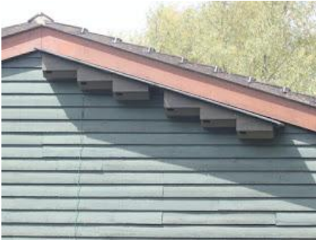
Boxes fitted to sloping fascia
