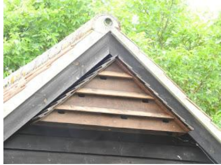
Boxes fitted to gable apex
