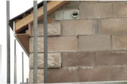
Schwegler 1A during installation at Sedbergh People's Hall
